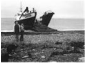
2003.046.0076 Barge and equipment at English Bay.
